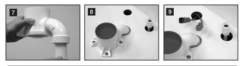
IMPORTANT: Do not attempt to slide the toilet over the discharge adapter. The toilet must be set down into the adapter to prevent possible damage.
