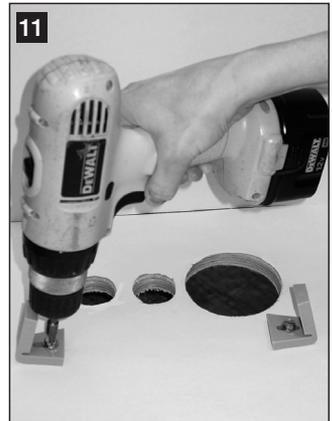
6. Use Dometic DFT touchpad template to mark location of fastener and access holes. Drill 1 in. (25 mm) hole, then fasten panel bracket to wall (fig. 12).
