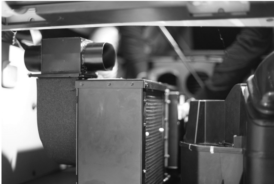
Figure 4: Plenum Installed on CHEB Blower
