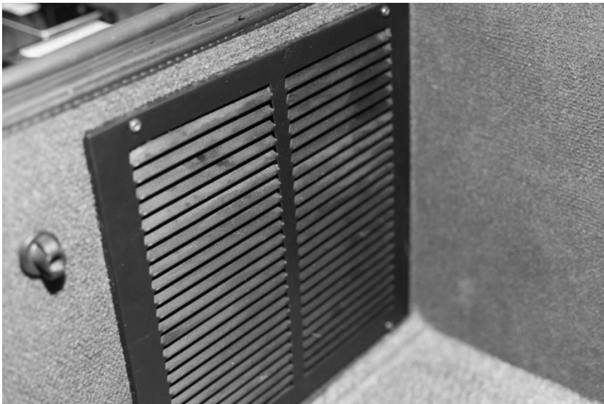
Figure 11: Return Air Grille Installed Near CHEB
