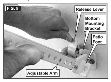
2. A WARNING IMPACT OR CRUSH HAZARD. Anchor patio foot securely when placing awning in carport position. Otherwise, product may become unstable and could [detach / bend / collapse]. Failure to obey this warning could result in death or serious injury.
